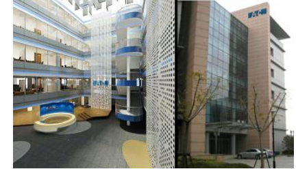
Eaton Regional HQ (Shanghai, China)
