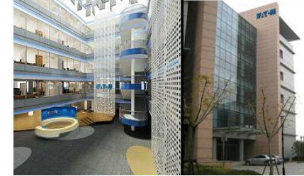
Eaton Regional HQ (Shanghai, China)
